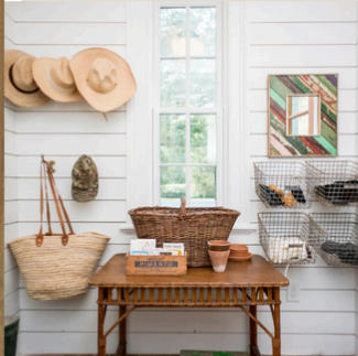
SHIPLAP ON WALL OPPOSITE BUILT-INS
